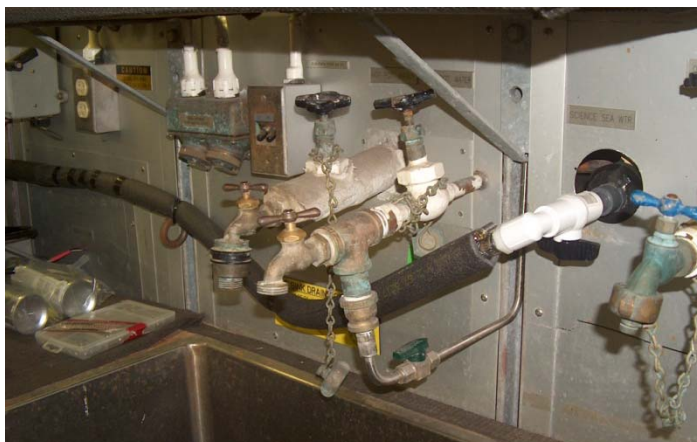
Figure 8: Seawater source valve, with insulated tubing leading to equilibrator.
