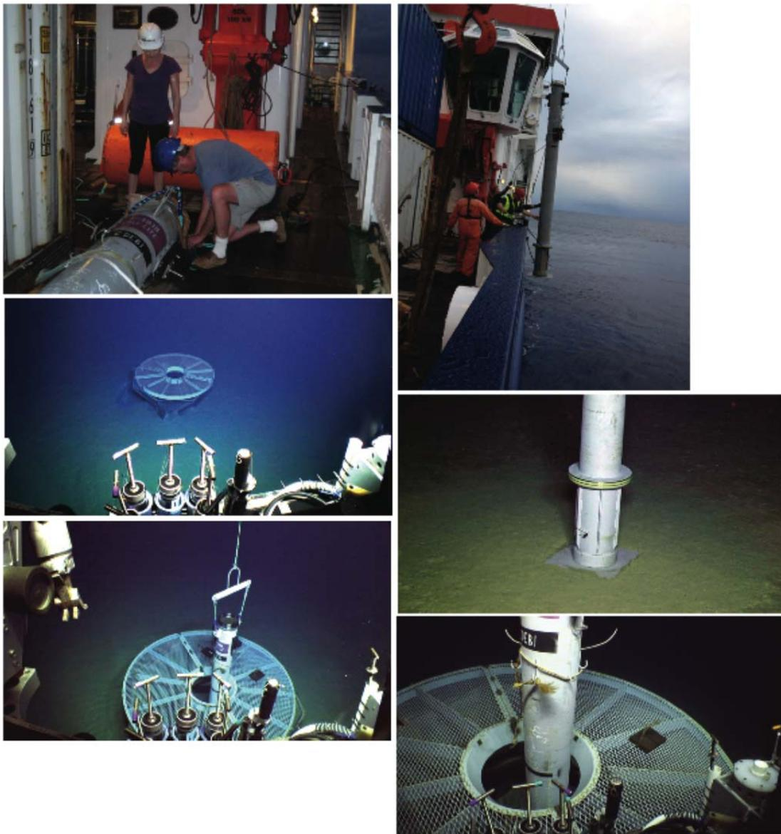
**Fig. 5.6** Preparation, launch and installation of the CORK lite in Hole U1382A
